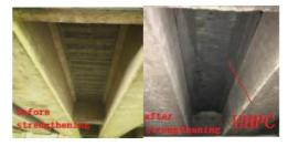
Fig.3 the effect drawing of UHPC
